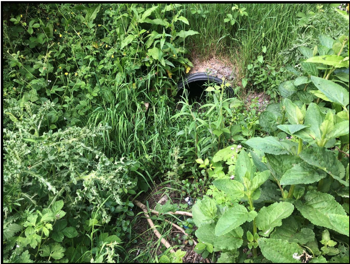
Plate 3.10 Image of a drain adjacent to the stream to the west
