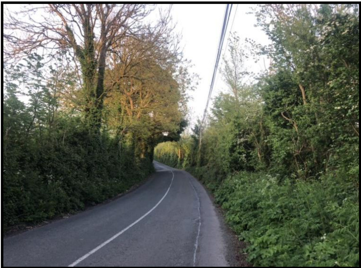
Plate 3.6 Looking east along the existing road
